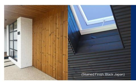
This Thermory® cladding and lining profile is designed specifically for the Australian market and available exclusively through City Timber. Featuring Thermory's hidden fixing system and end matching for fast installation, the Trax design features a contemporary, linear ribbed profile, plus the benefits of a thermally stabilised timber. With increased dimensional stability and durability, the Trax profile is designed to perform in Australian conditions.
