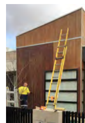
STAINING: Stain in the same direction that the boards run eg. Vertical for vertical cladding.
